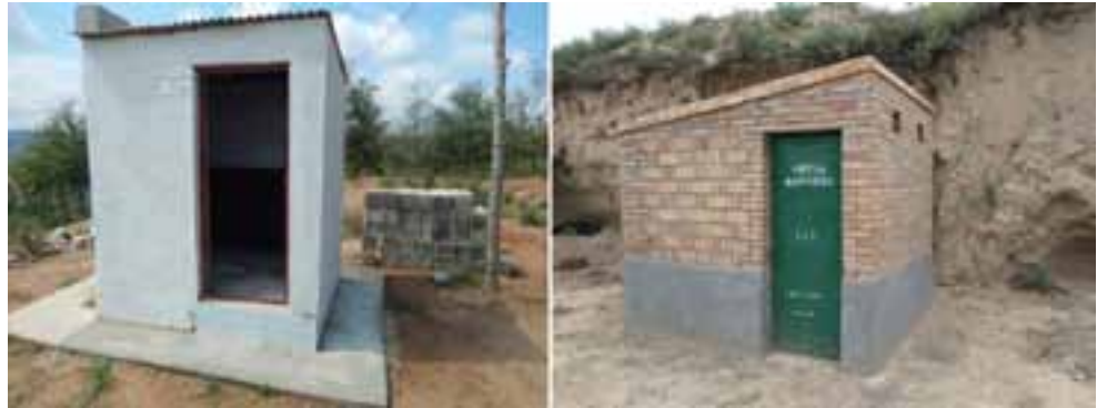
建成的砖木结构卫生旱厕 / post and panel structure toilet
